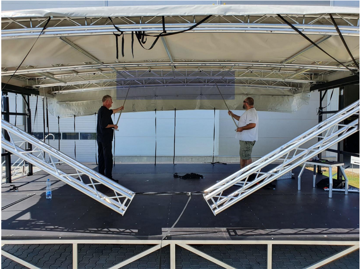
Photo: Roof stiffness bar (a)
